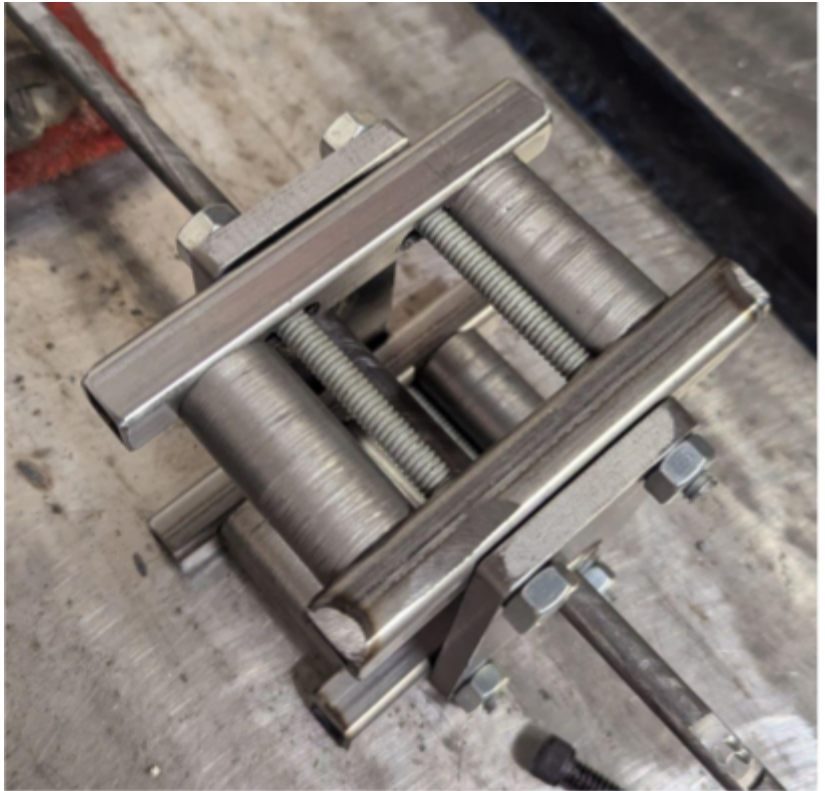
Figure [23]: The gearbox frame bolted into its frame prior to welding
